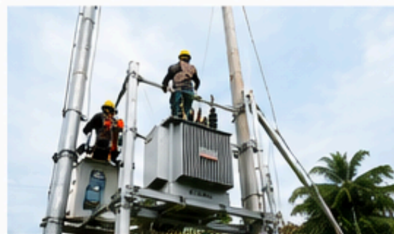
INSTALASI TRANSFORMATOR
